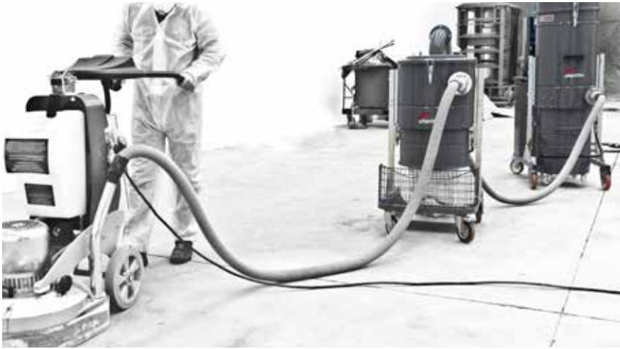
Separators with Longopac discharge system for floor preparation
